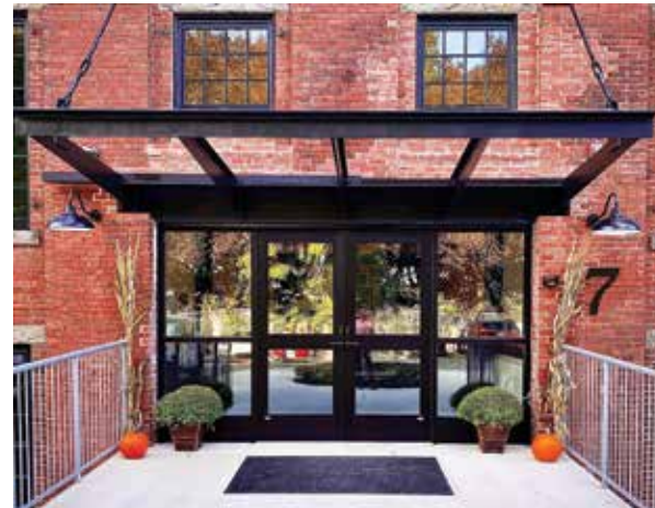
Entrance to The Lincoln Hotel. Courtesy photo.
